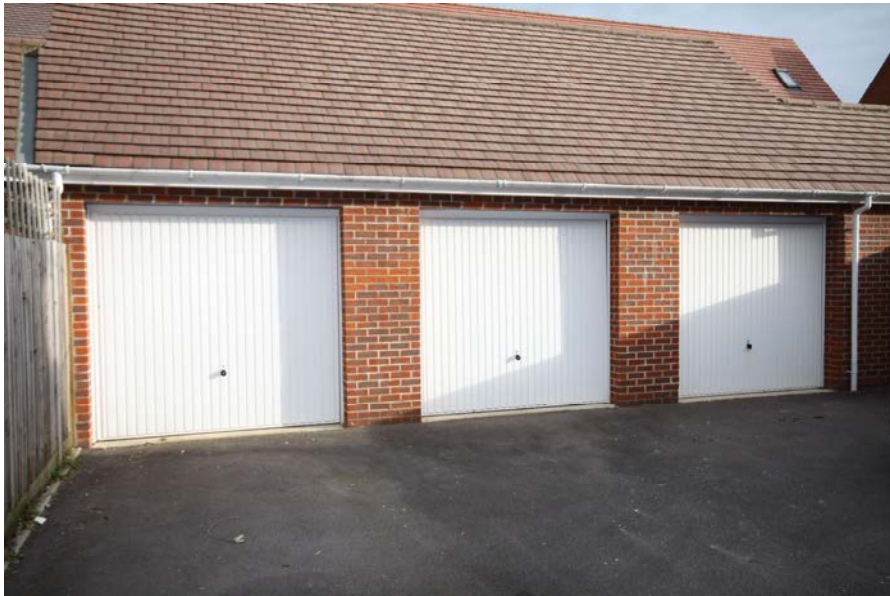
Garage in block
